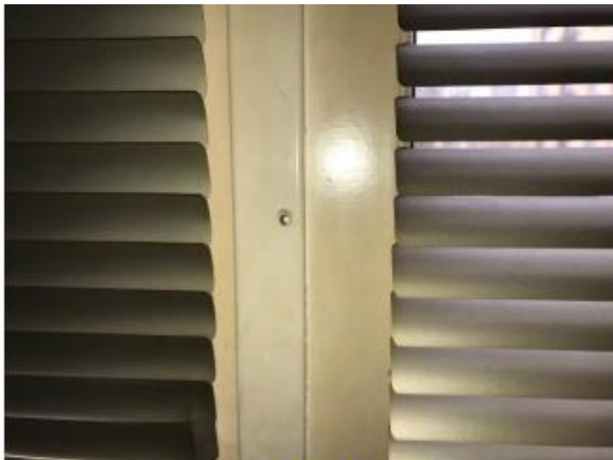
Fitment holes to doors
